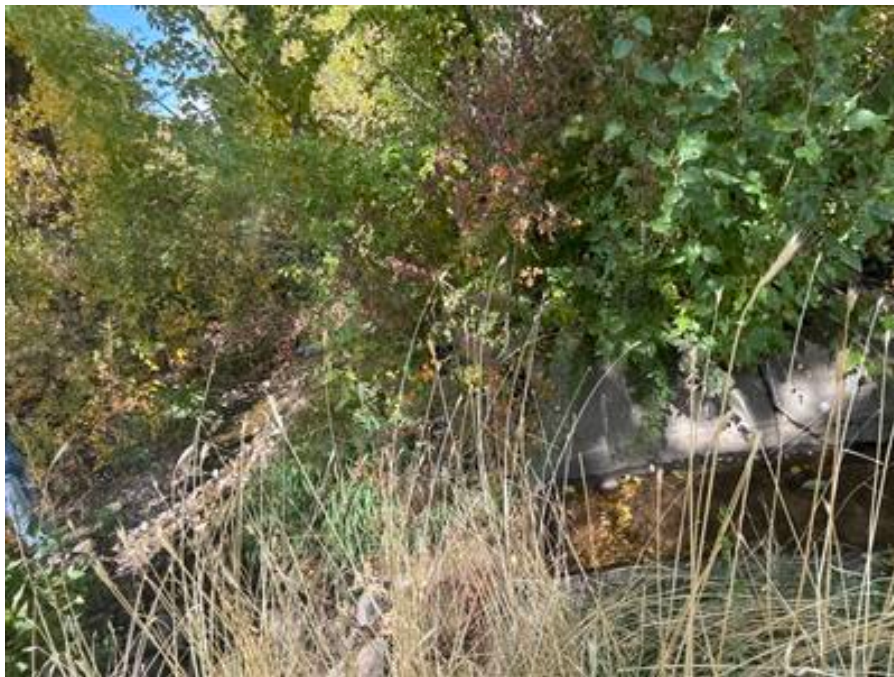
Photo of ditch D-1 (location shown in Attachment B, page 17).
