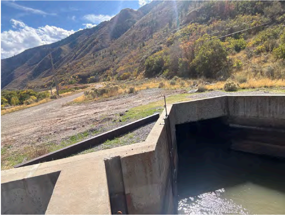
Upstream View (Date: 10/13/2025)
