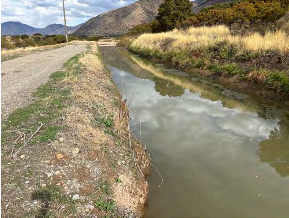
Upstream View (Date: 10/13/2025)
