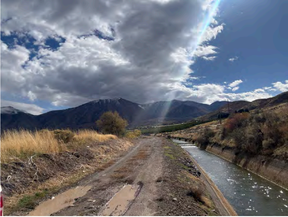
Upstream View (Date: 10/15/2025)
