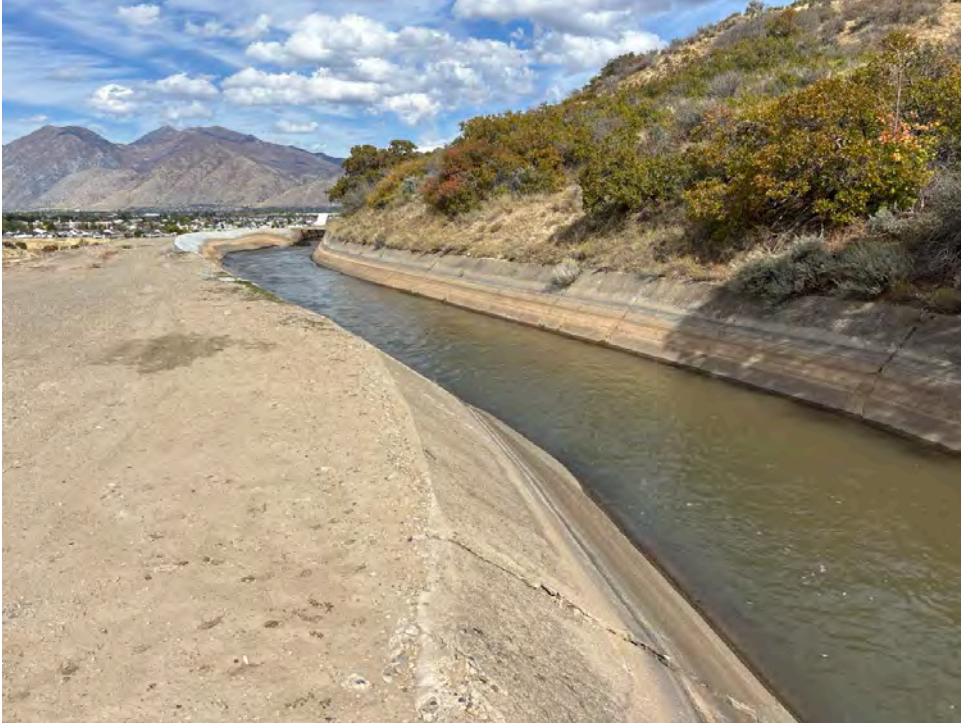
Upstream View (Date: 10/13/2025)
