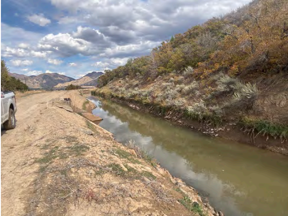
Upstream View (Date: 10/13/2025)
