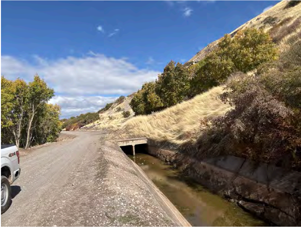
Upstream View (Date: 10/15/2025)
