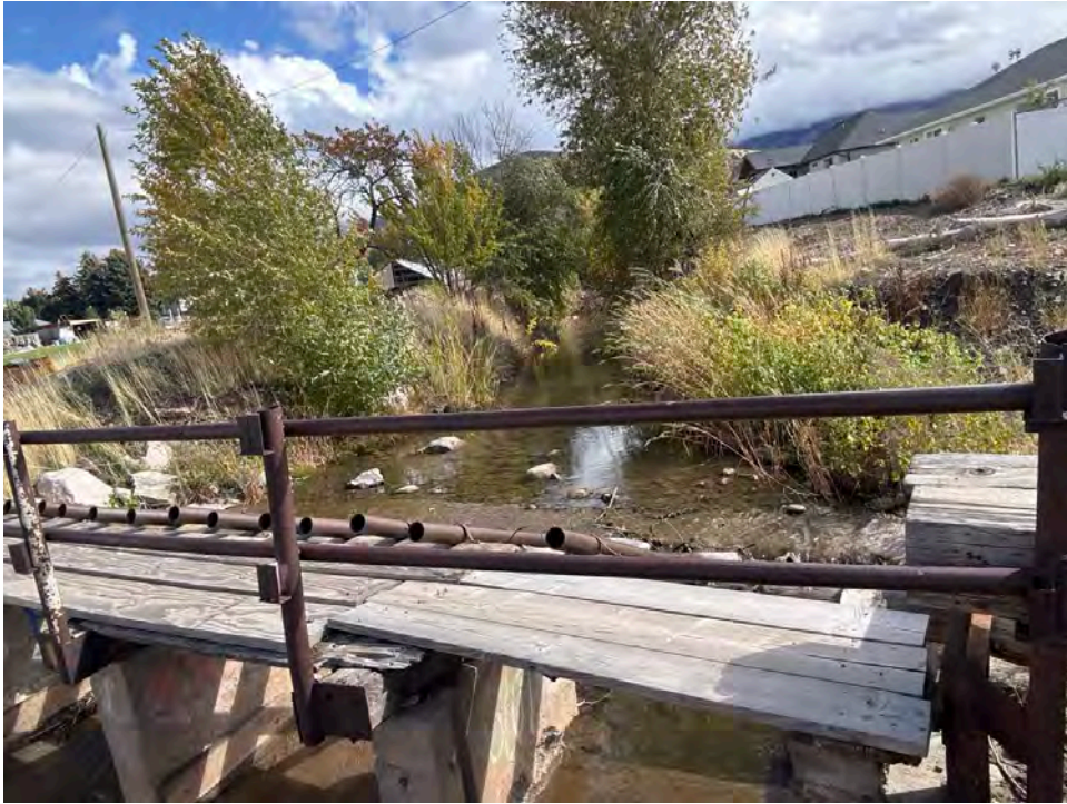
Upstream View (Date: 10/15/2025)
