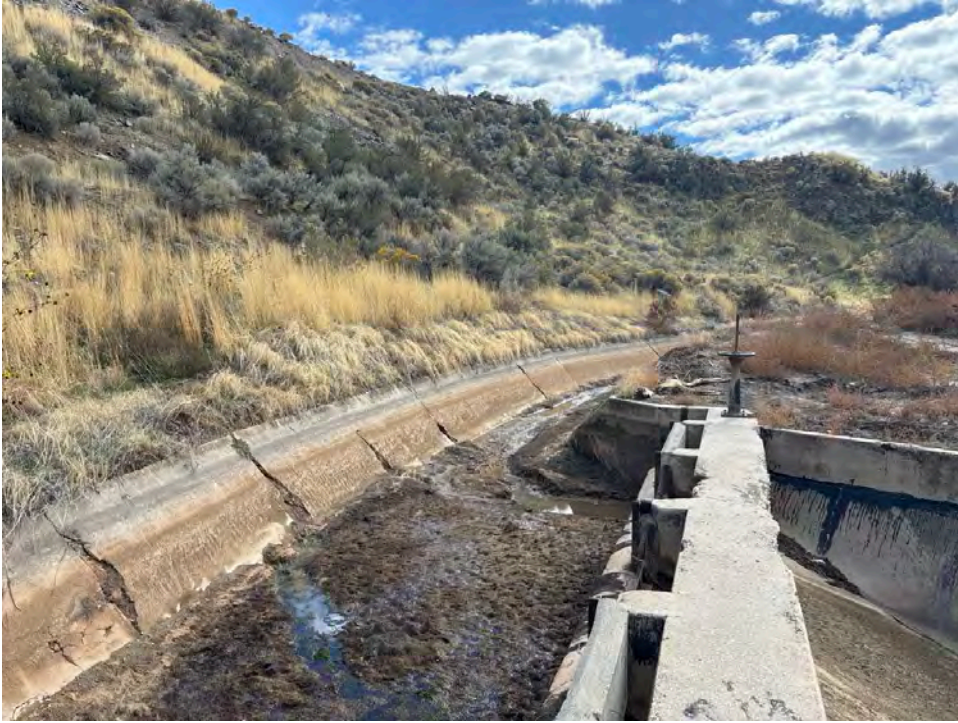
Upstream View (Date: 10/16/2025)
