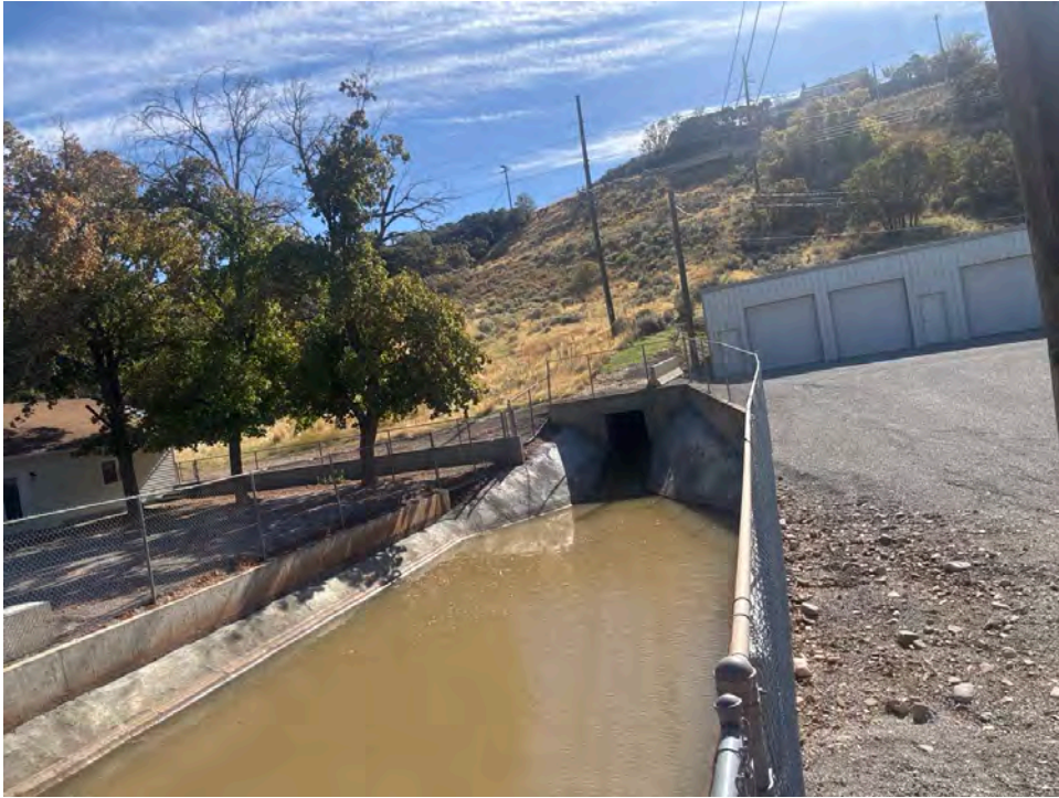
Upstream View (Date: 10/13/2025)
