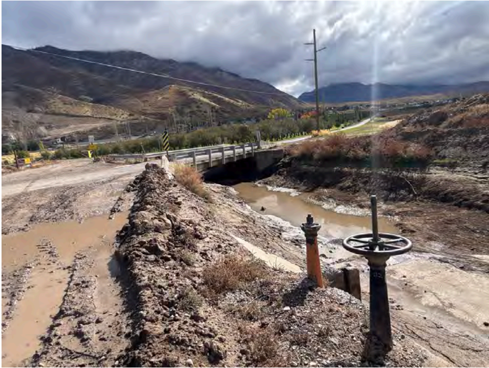
Upstream View (Date: 10/15/2025)
