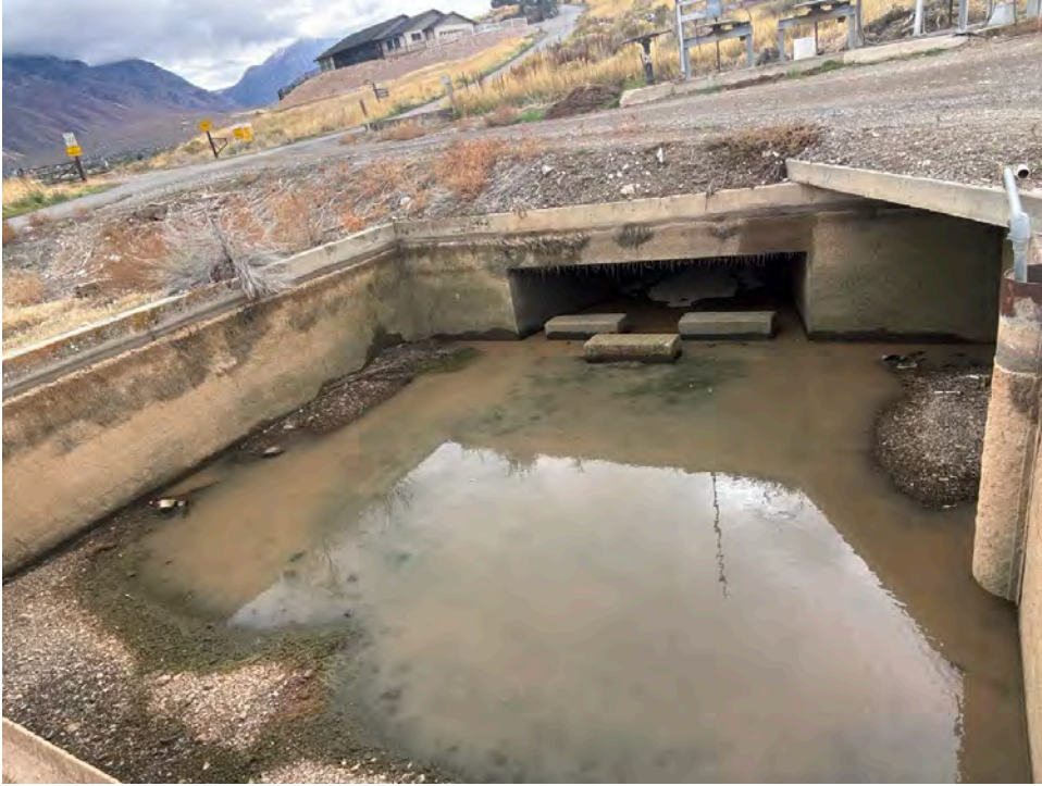
Upstream View (Date: 10/15/2025)
