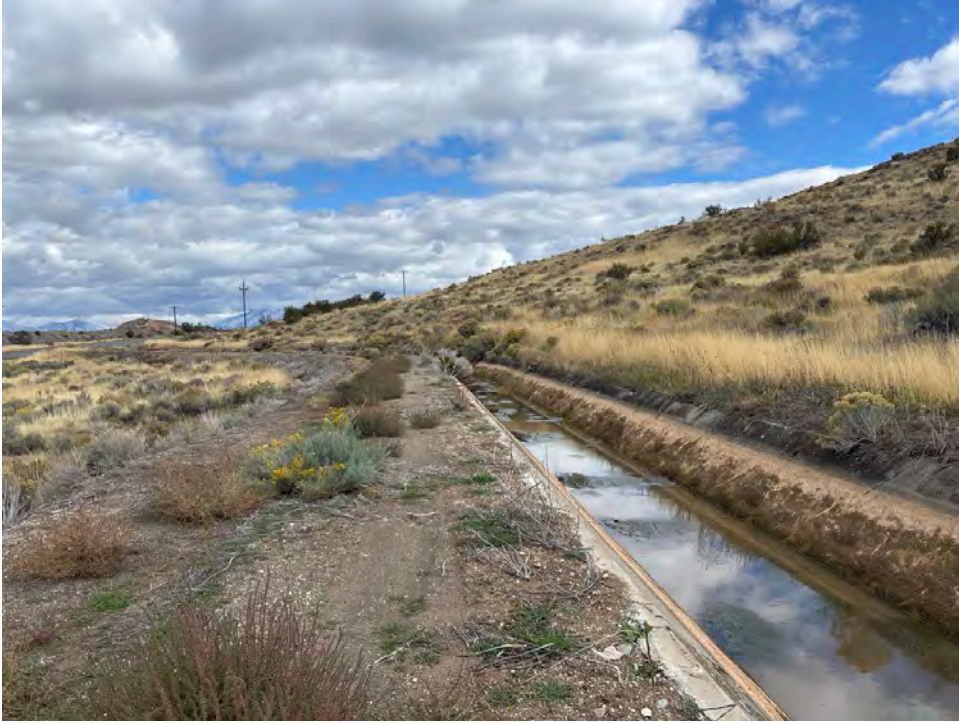
Upstream View (Date: 10/16/2025)
