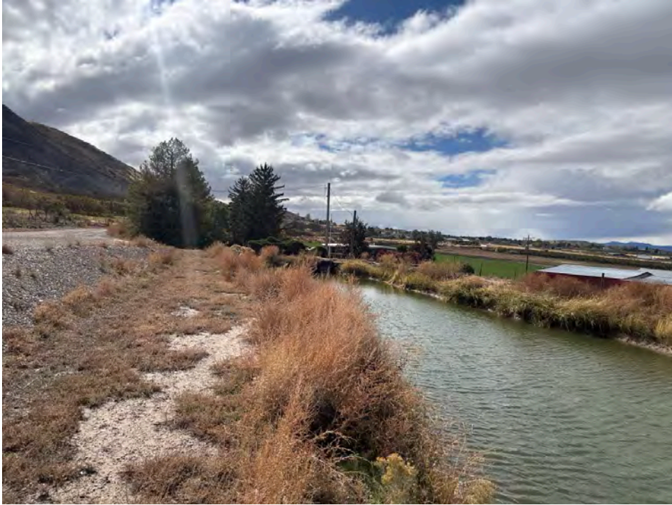
Upstream View (Date: 10/15/2025)
