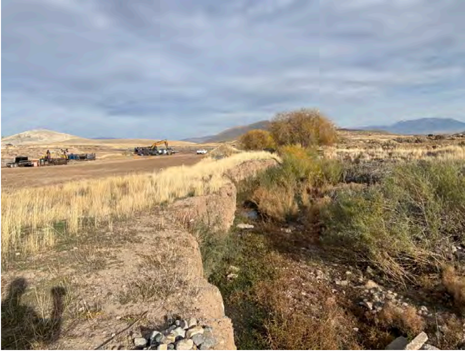
Upstream View (Date: 11/5/2025)
