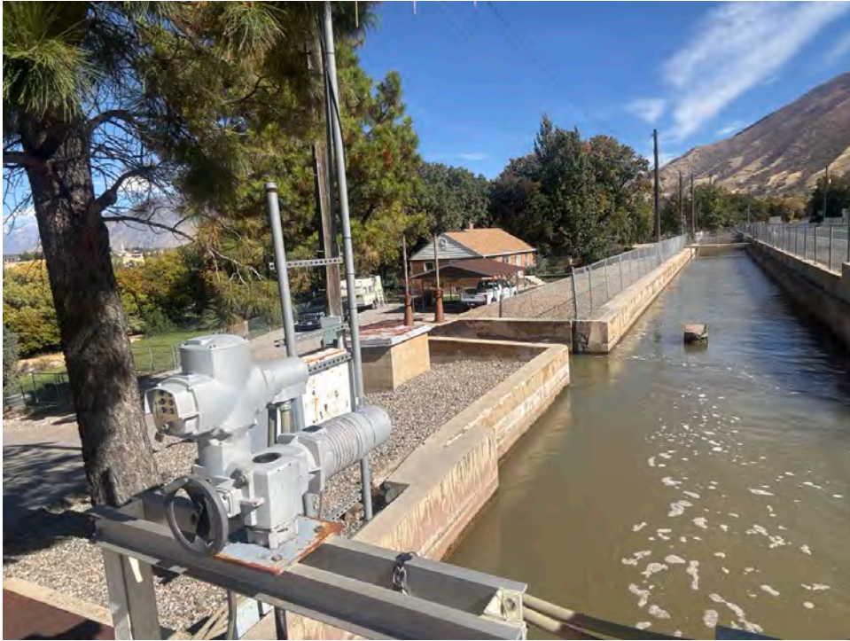
Upstream View (Date: 10/13/2025)
