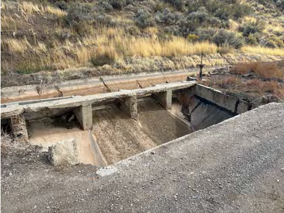
Upstream View (Date: 10/16/2025)
