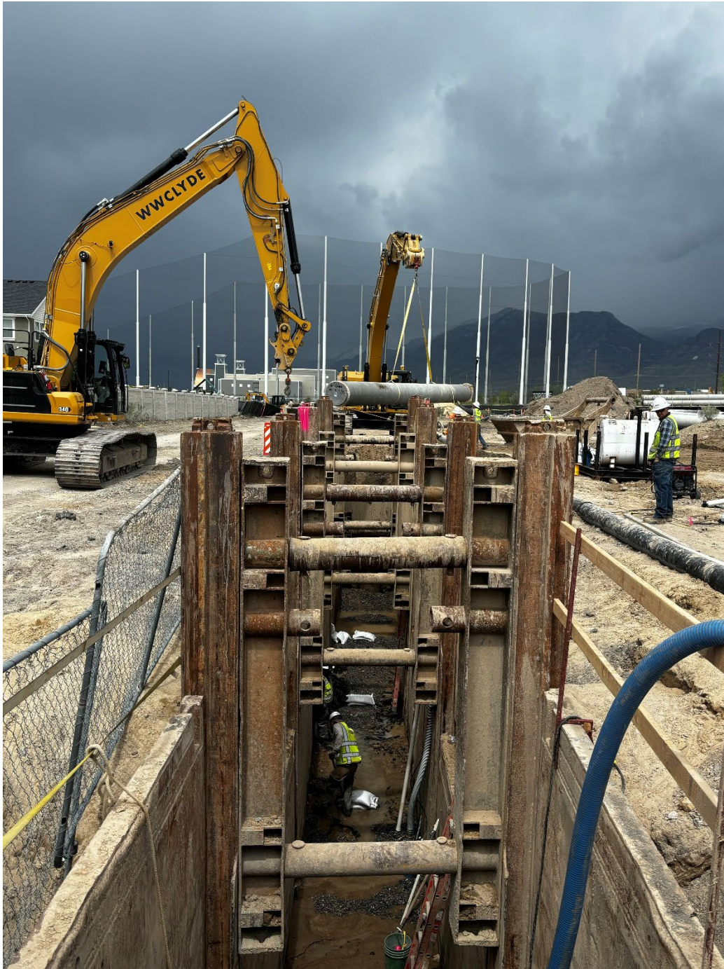
Welded Steel Pipeline Installation
