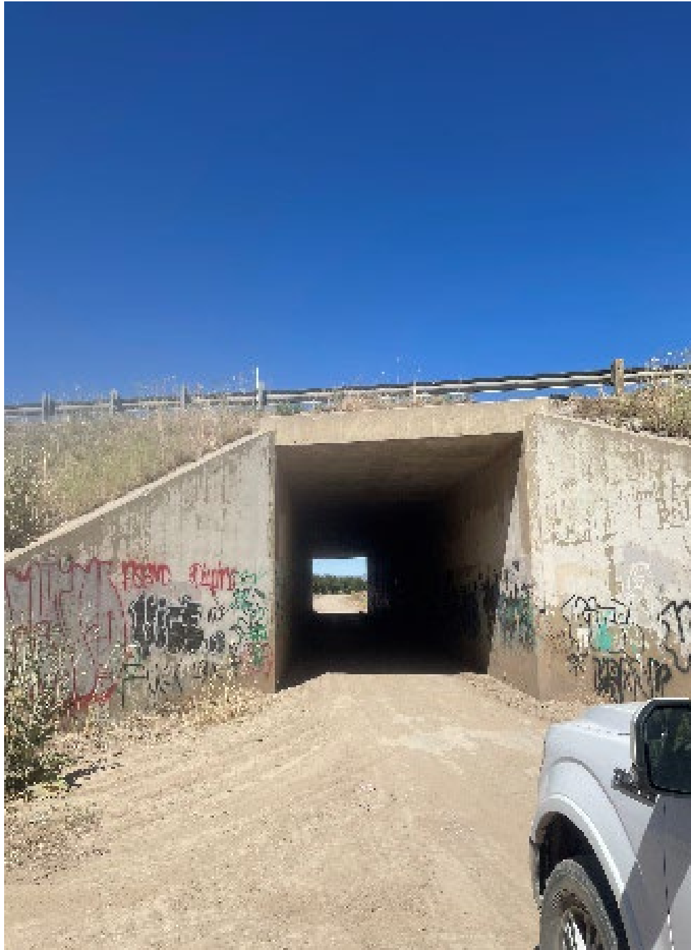
Existing Truck Tunnel Under I-15
