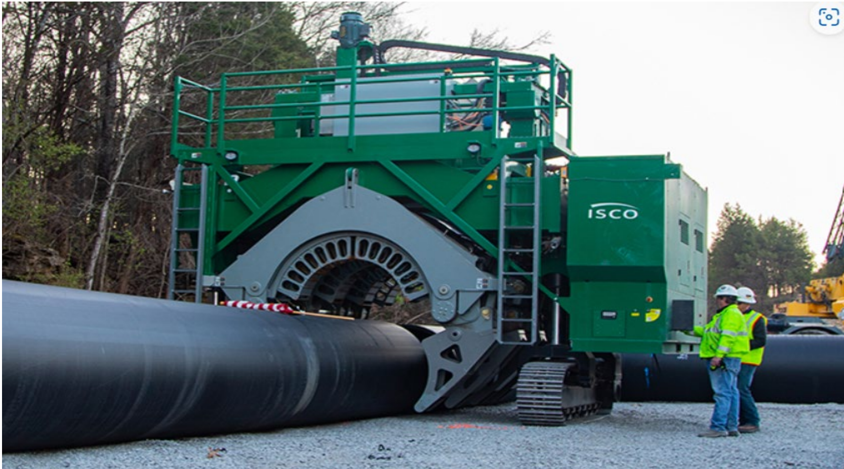
Large Diameter HDPE Pipe with Fusion Machine
