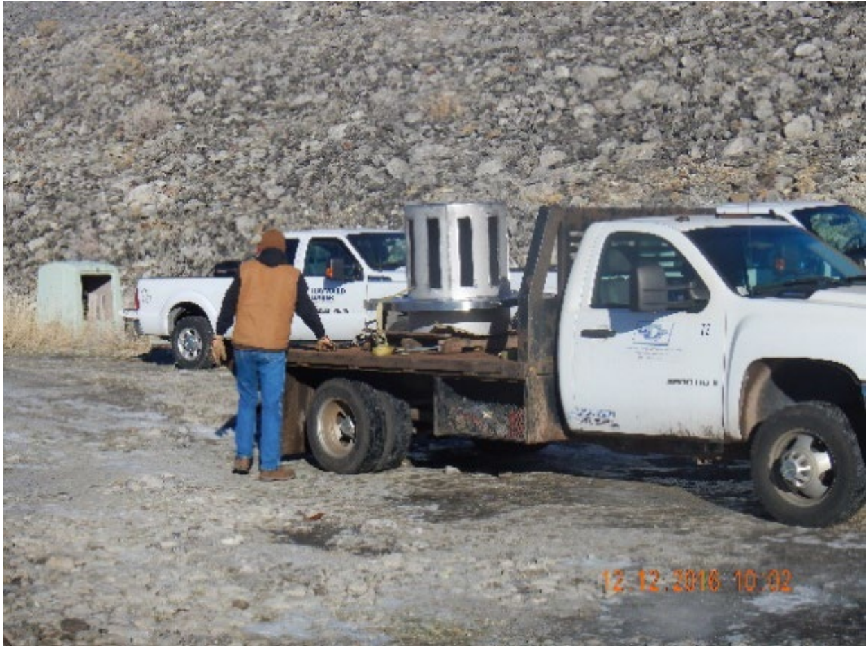
Energy Dissipator Arriving On-Site
