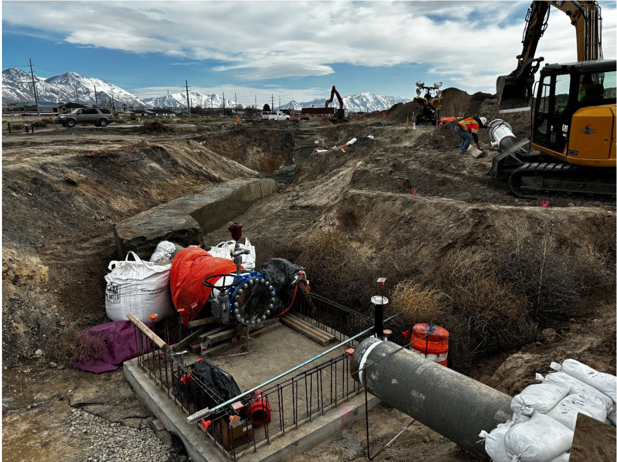
20-Inch Double Offset Butterfly Valve
