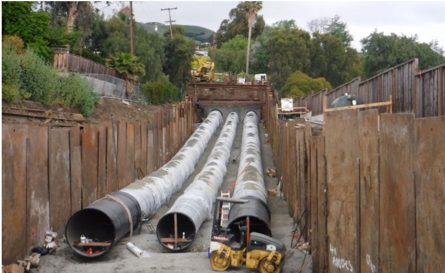
ERDIP Installation in Earthquake Prone Santa Clara Valley, California
