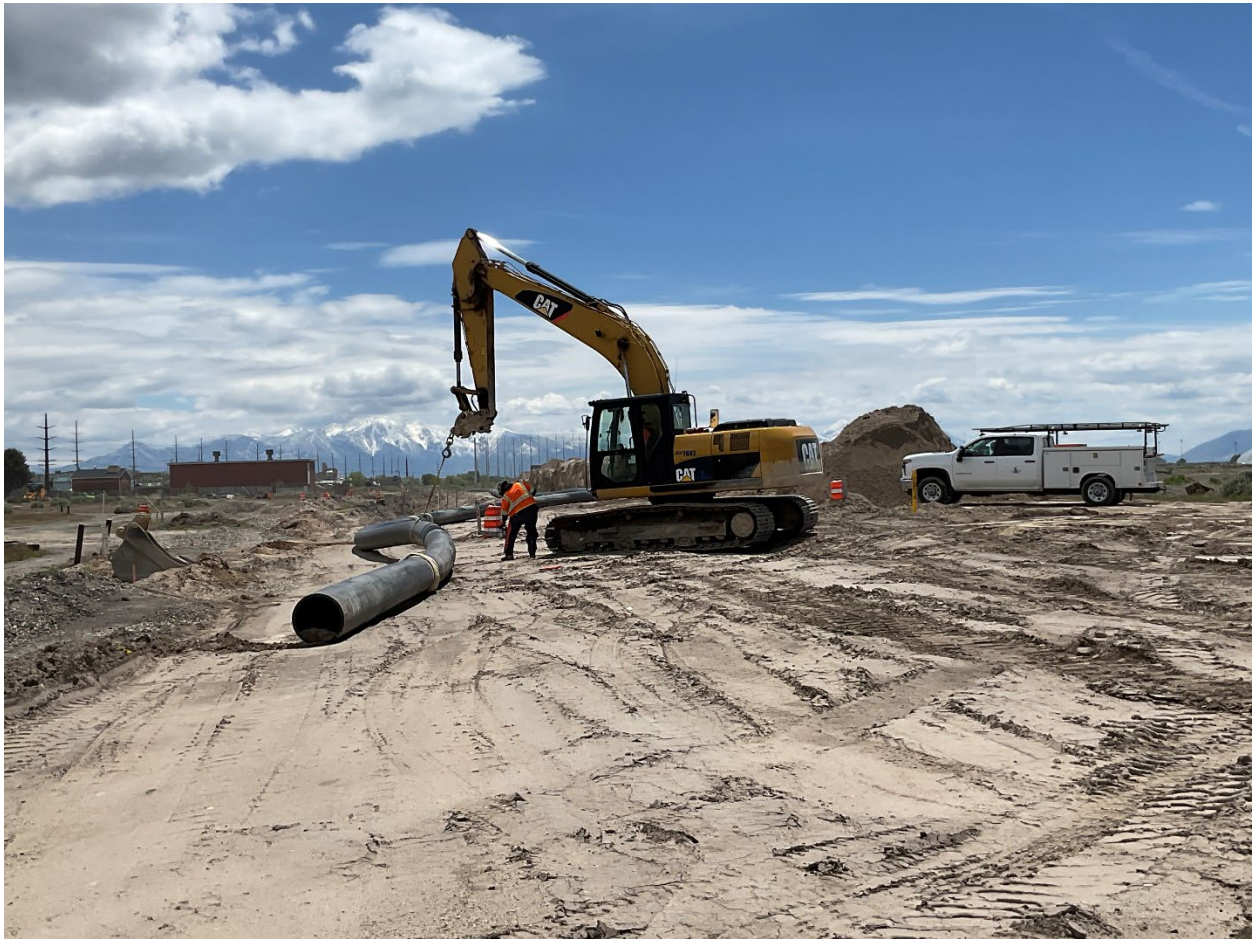
HDPE Pipeline Installation
