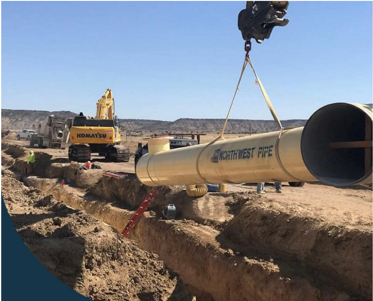
Typical WSP for Water Transmission
