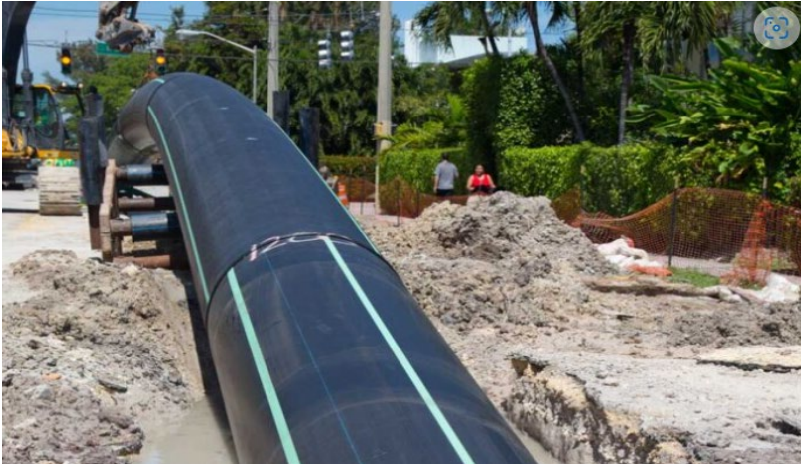
Large Diameter HDPE Pipe Installation Example
