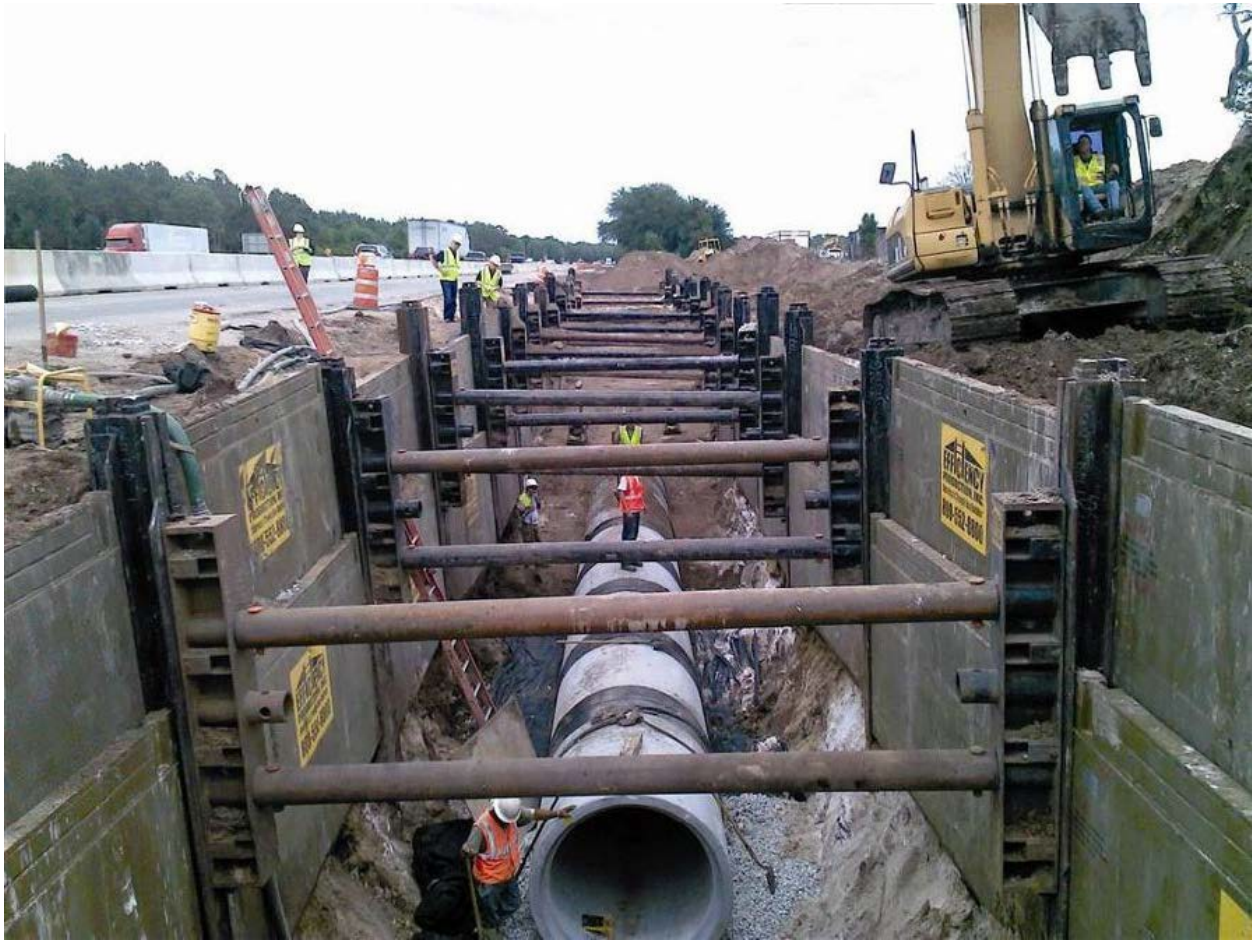
Conventional Pipeline Backfill
