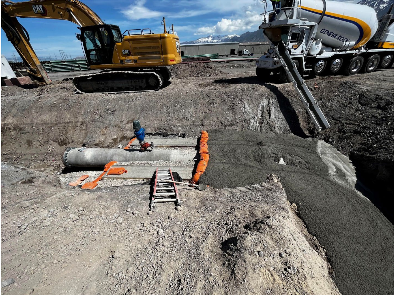
Photo of CLSM Backfill
