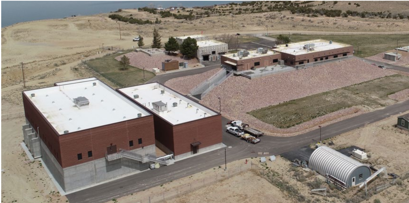
External Stairs and Stairs Up Steep Slopes Complicate O&M Access at the Duchesne Valley WTP The Alternative Grading Plan Eliminates these Issues.
